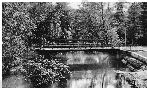
North Avenue Bridge
