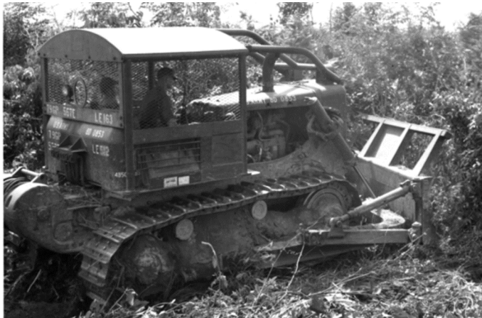
The Rome plow, the Army Engineers marvel, introduced in 1967. With its razor sharp blade, a team of 30 could clear 200 acres of dense jungle in a day. A landing zone or air strip could be created in days where before it would take weeks.
