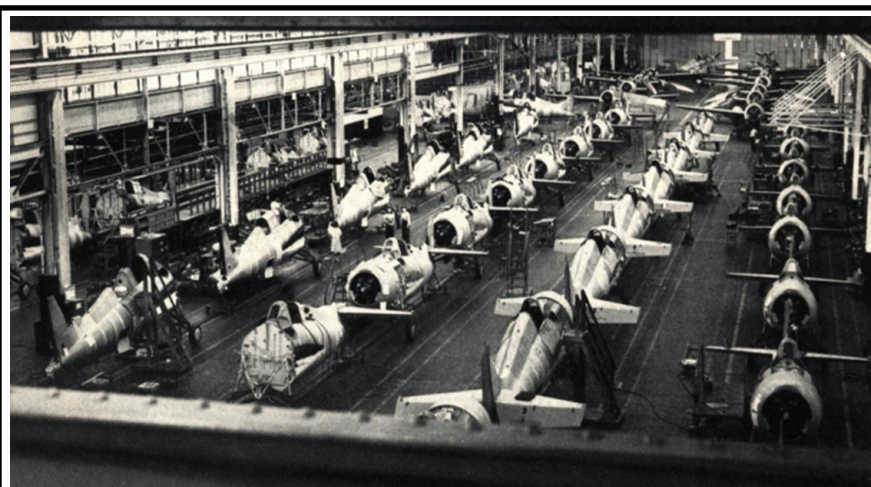
Assembly lines at Linden's Eastern Aircraft, formerly General Motors. 35,000 Wildcats and Avengers were assembled in Linden and Trenton by 1945.
